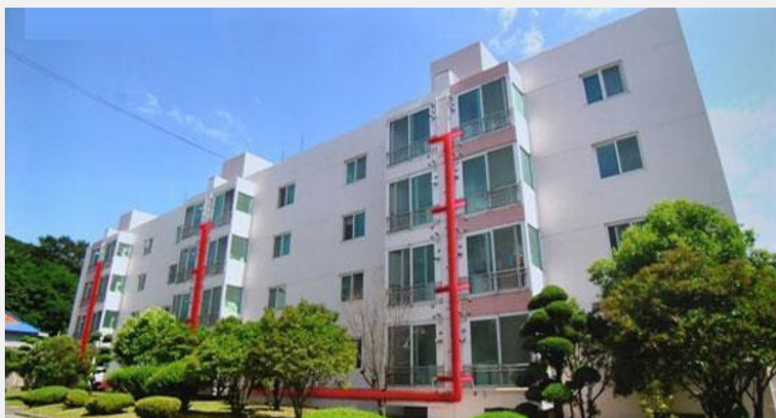
Figure 50 Hydrogen pipelines (red) installed on the external wall of the apartment (Shin, 2014)
