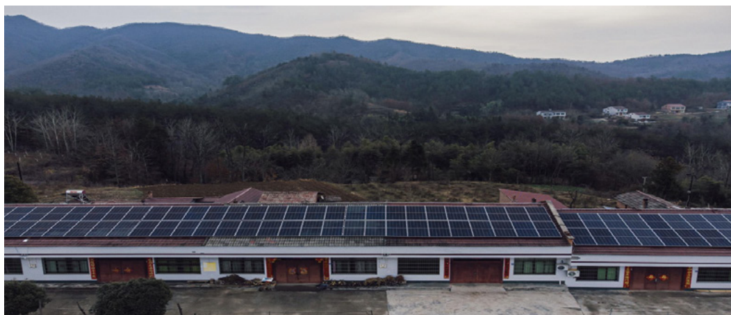
Figure 16: Installation of Solar Panel in Hanyin County.
