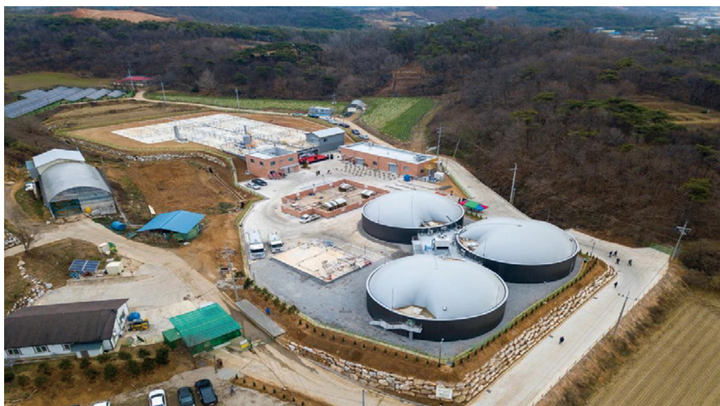
Figure 31: Aerial View of Biogas Plant.
